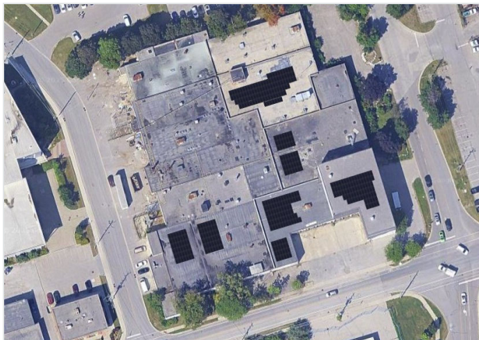
Site A, Ajax, ON — the largest of the three: 611 kWdc across nine roof sections
